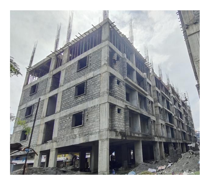
**Block B1:** External plastering work –South Side elevation 100% completed, East side elevation 40% completed, West side elevation 25% completed, South side elevation 10% completed.
