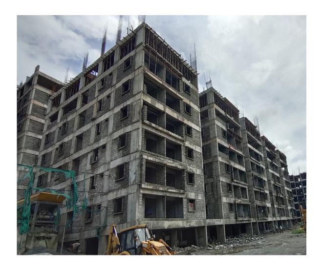
**Block D1:** Ninth Floor level slab Concrete casting 100% completed. Shuttering works for 1<sup>st</sup> half of Tenth floor level slab 10% completed.
