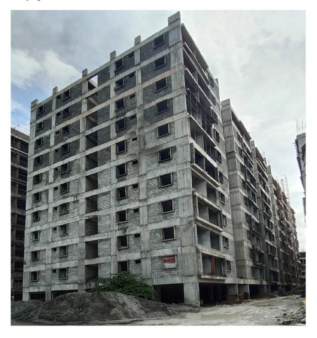
**Block C3:** Eighth Floor level slab 1<sup>st</sup> half Concrete casting 100% completed. Shuttering works for 2<sup>nd</sup> half of Eighth floor level slab 95% completed and balance works on progress.
