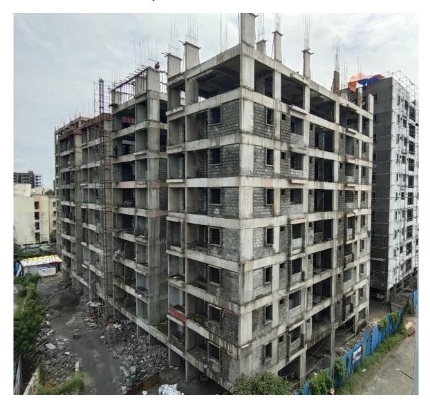
**Block D2:** Terrace Parapet Columns concrete 100% completed. External Plastering work in West side elevation 100% completed, North side & South side elevation 10% completed.
