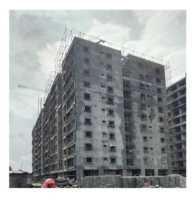
**Block C2:** Terrace floor level slab 100% completed. Shuttering & Reinforcement for Lift Base slab on progress
